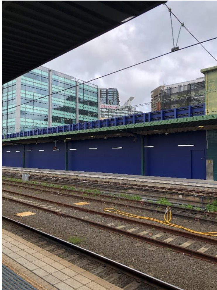
Figure 1-20: Platform 1 A-Class Hoarding
