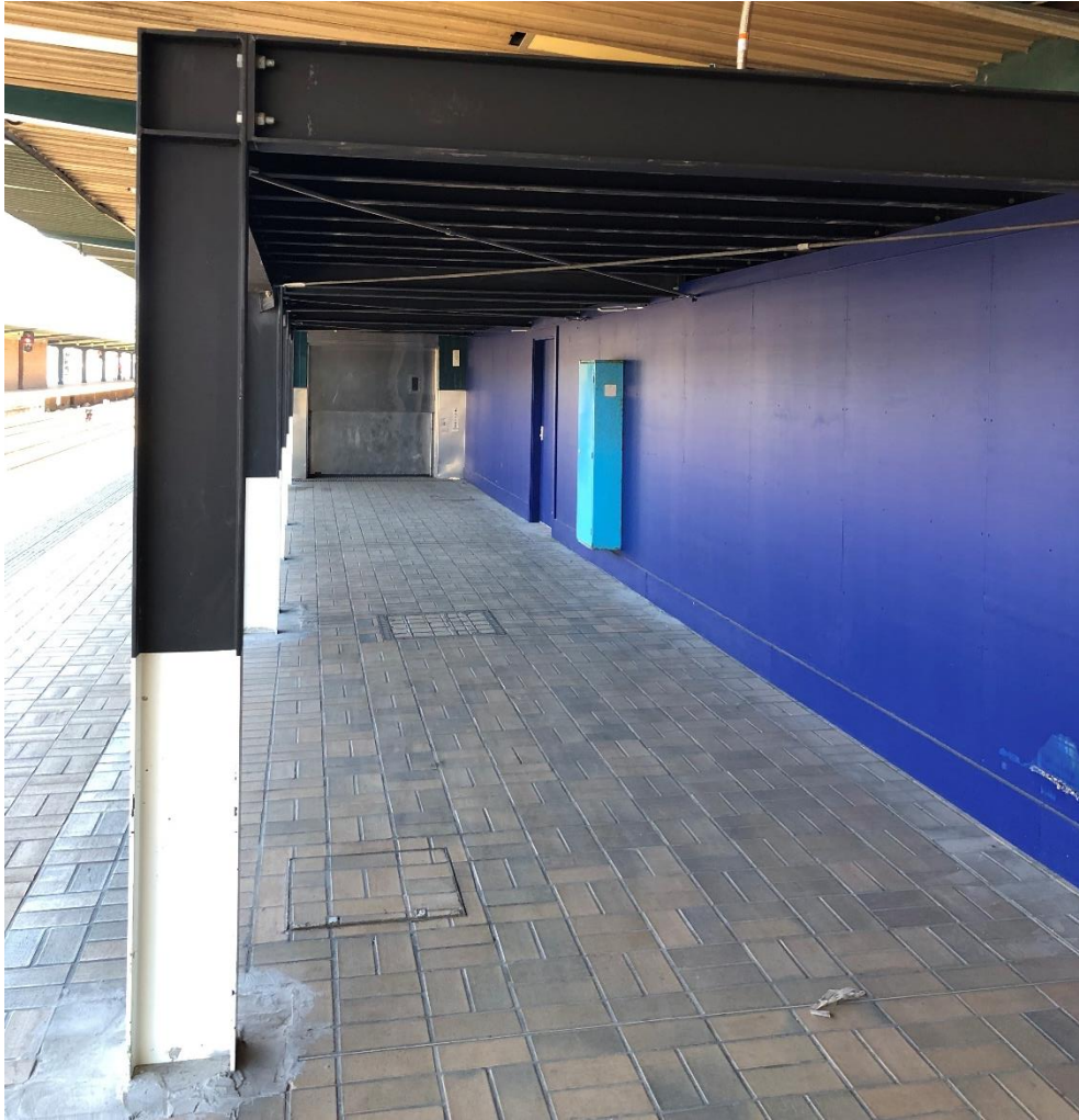
Figure 1-13: Platform 1 B-Class Hoarding
