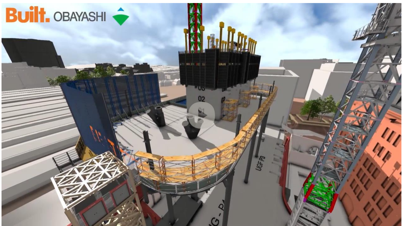
Figure 1-48: YHA Edge Protection (Model Depiction)
