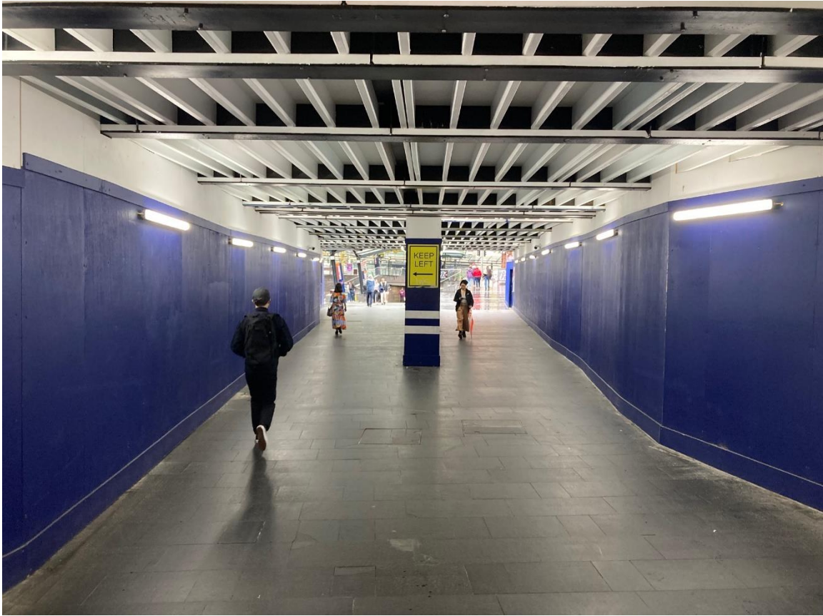
Figure 1-17a: B-Class Hoarding – Devonshire St Tunnel
