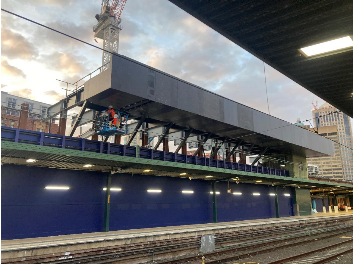
Figure 1-45: View of the Platform 1 Overhead Protection Deck facing West
