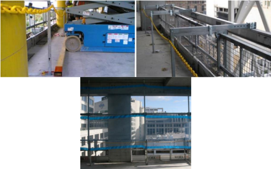
Figure 1-54: Photographic Example of WorkRight Edge Protection System inc. Netting
